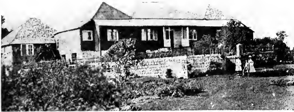
Typical planter's house. The three roofs are a protective device against high winds
